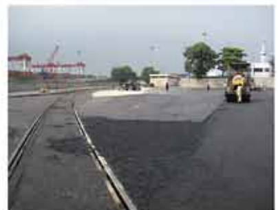
Extension of PACCS Yard
