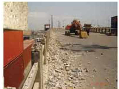
Old Bridge Dismantling
