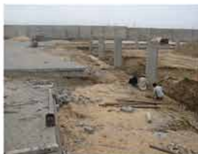
Northern Bypass ICD Construction
