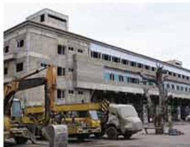
New Eight Lane Inner Gates and Gate House under Construction
