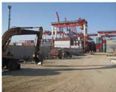
New Yard under Construction at Berth no. 5
