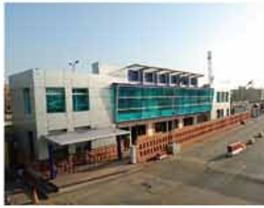
New Building Entrance at Gate
