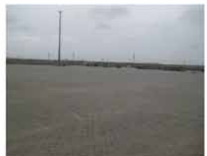
Northern Bypass ICD Construction
