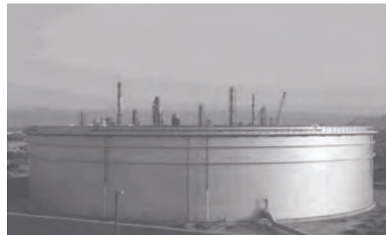
Byco takes pride in having the largest capacity crude oil storage tanks in the country.
