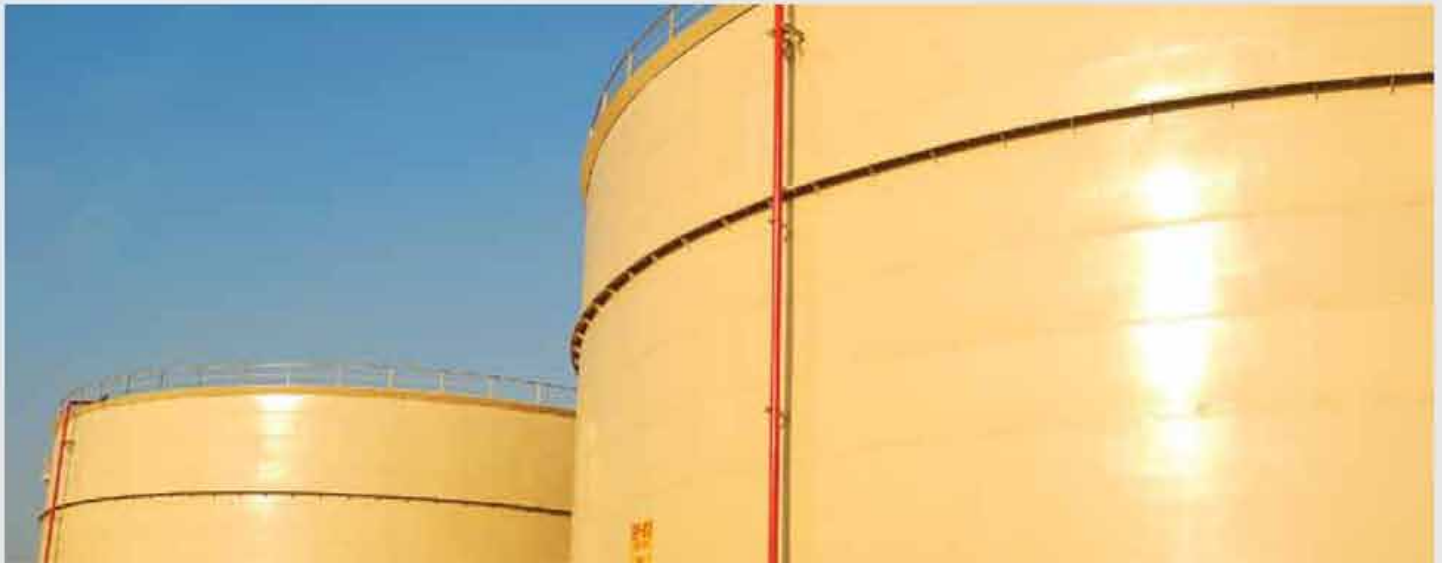
↑ The new tanks at Keamari were completed in December 2011 without a single safety incident.
