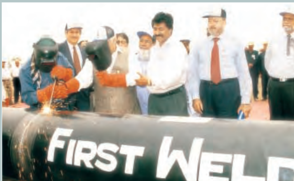
Sindh Minister for Mineral Development, Mr. Irfan Ullah Marwat, performing the first weld at the ground breaking ceremony of the 116 km, 24 inch Karachi-Hyderabad gas pipeline.
