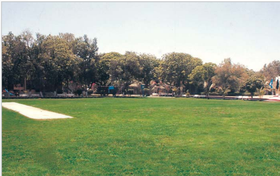
SOS Children Village Completed grassy play ground with seating for 200 children
