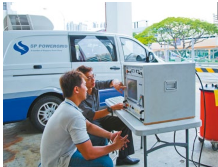
SP PowerGrid officers carry out an OWTS test in a substation.
