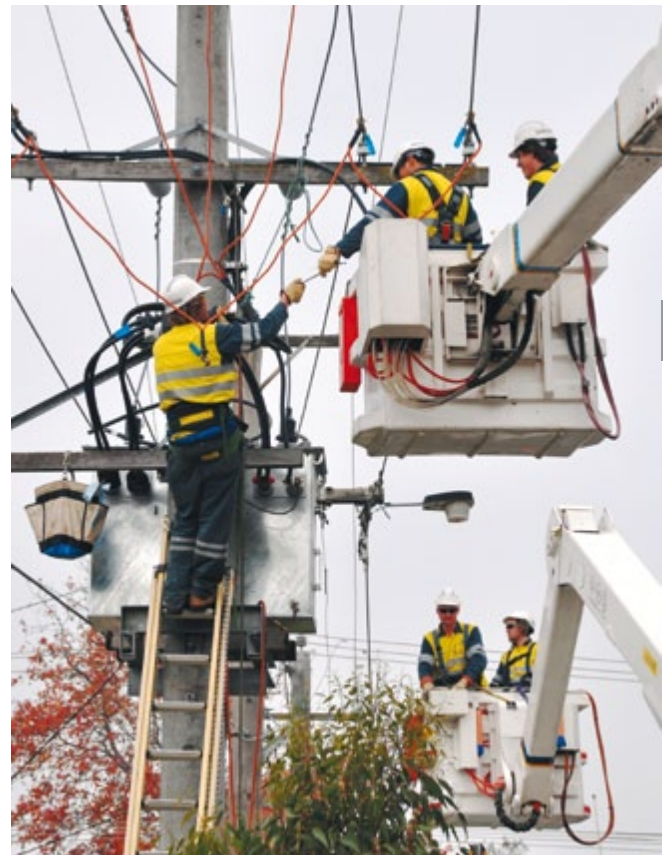
Replacing a pole in Melbourne.
