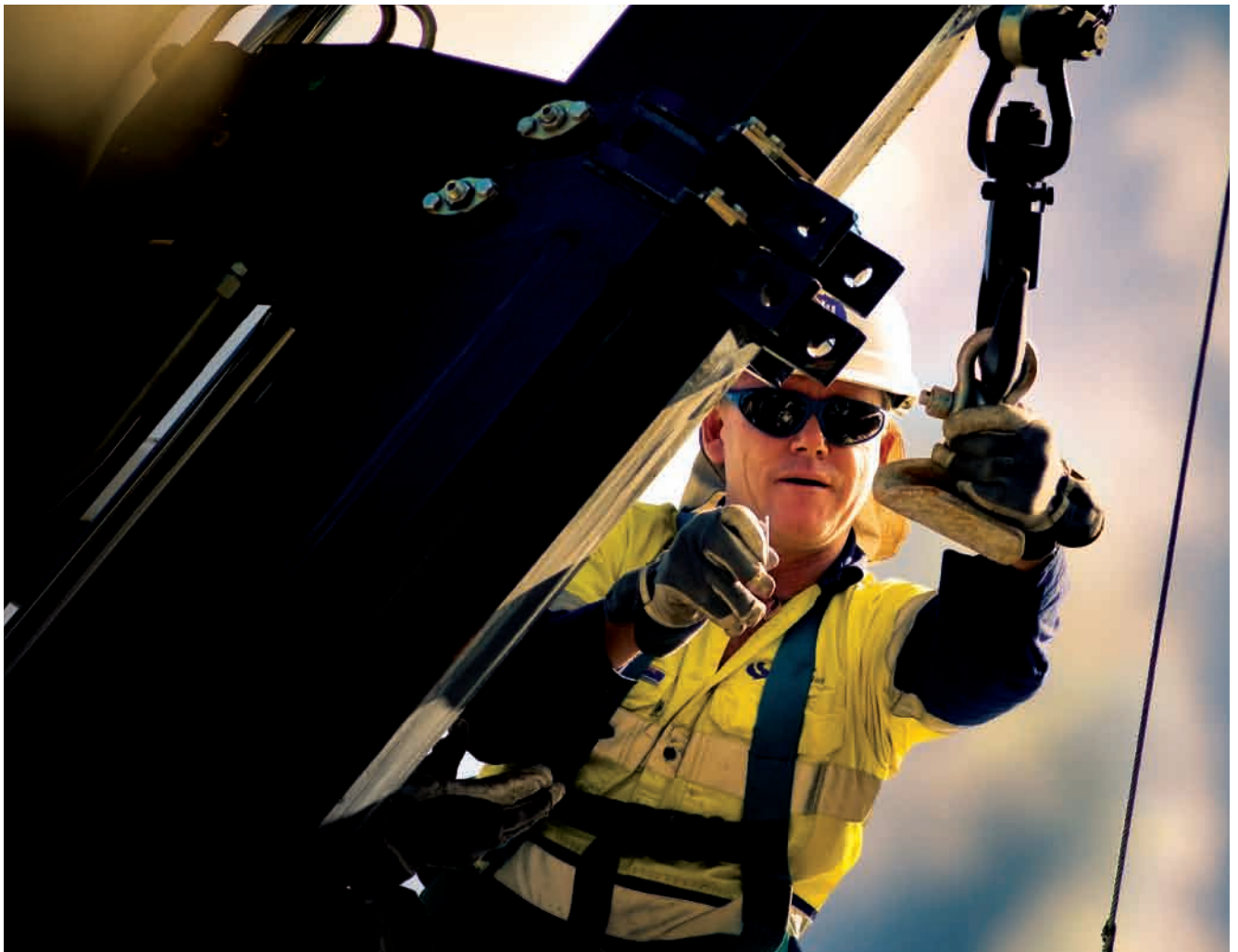
SP AusNet's electricity distribution network carries electricity from zone substations to customers in outer eastern metropolitan Melbourne and eastern Victoria.
