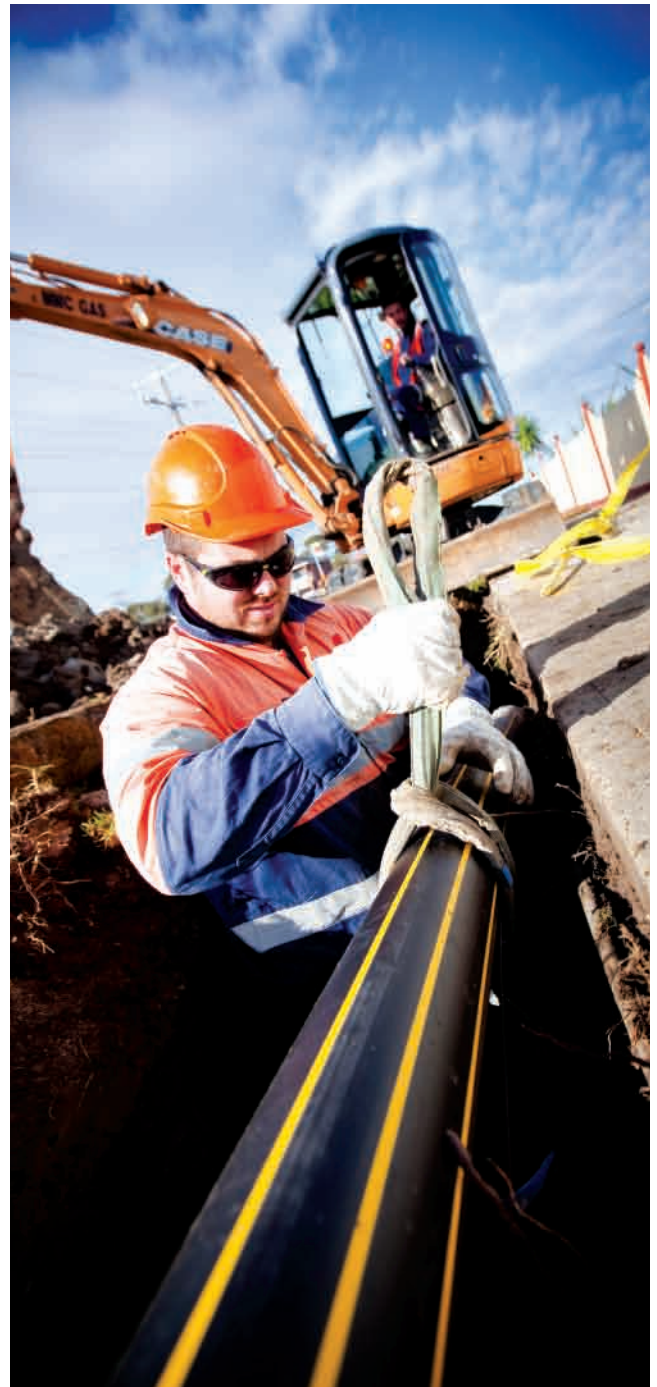
Gas distribution network installation in progress.
