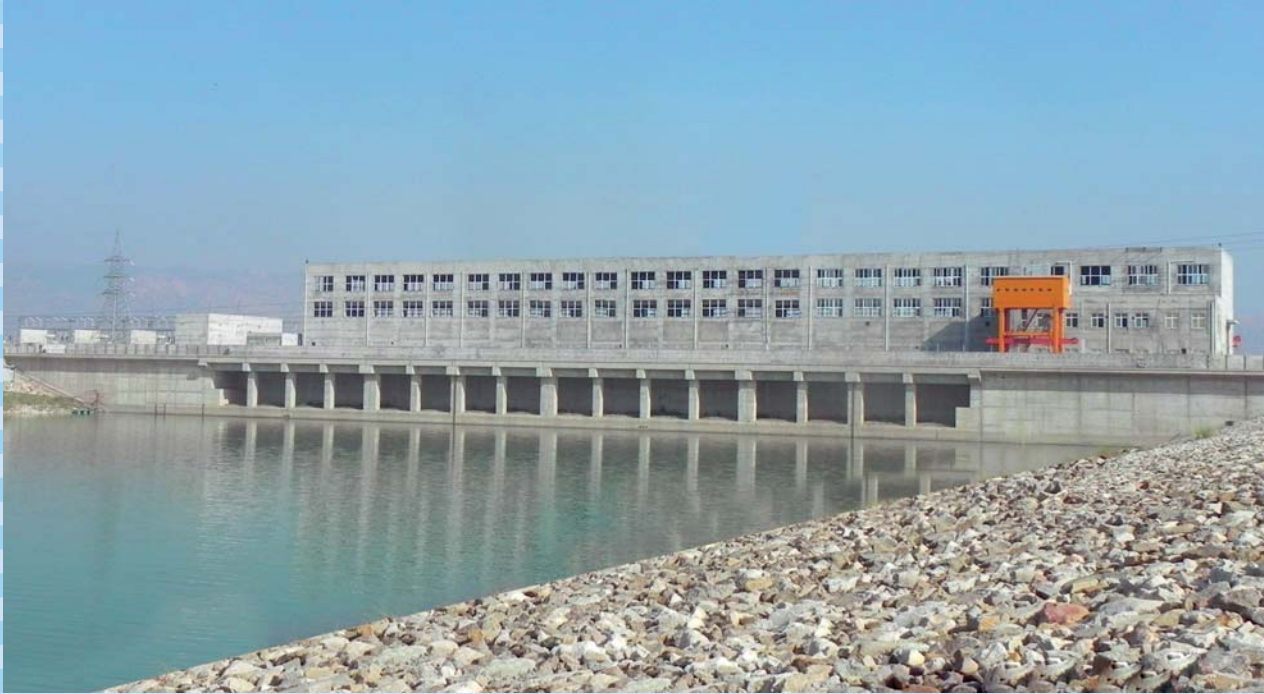
Down Stream view of Jinnah Hydrel Power Station
