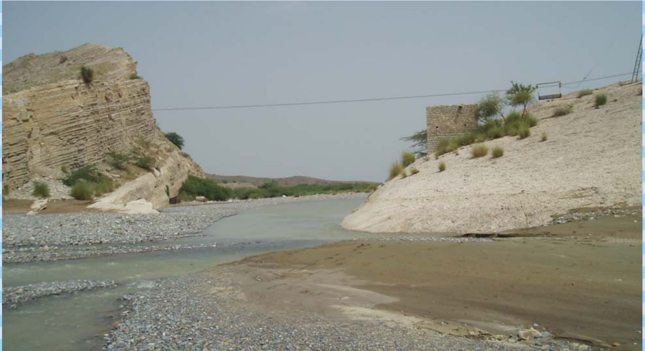
Site of Daraban Zam Dam
