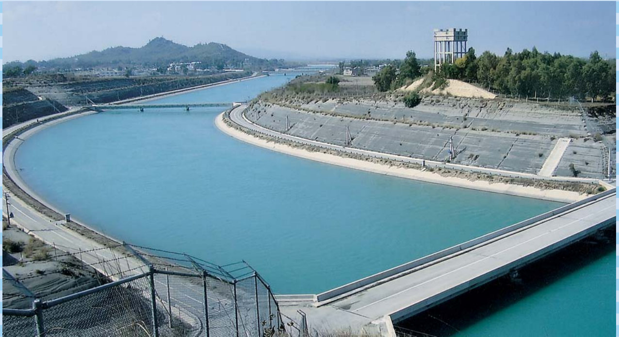
Power Channel of Ghazi Barotha Hydropower Project
