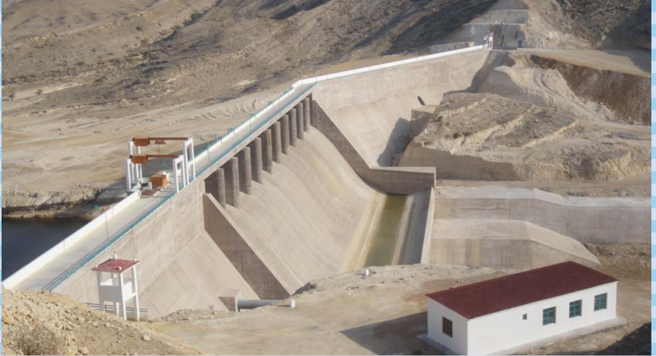
A View of Darawat Dam
