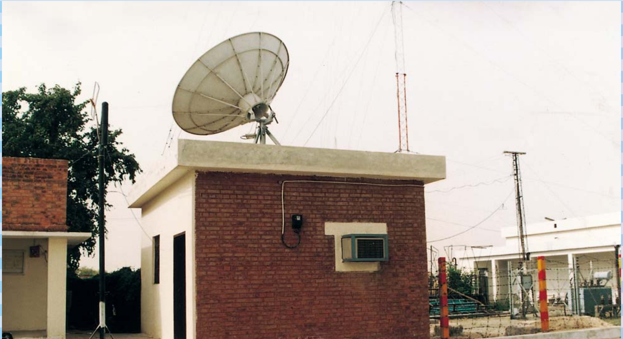
Control Room of Telemetry System at Chashma
