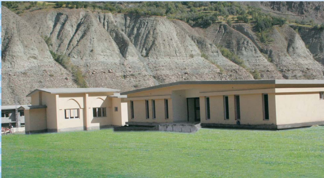
Golan Gol Project Offices
