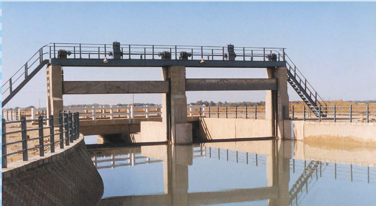
Chashma Right Bank Canal
