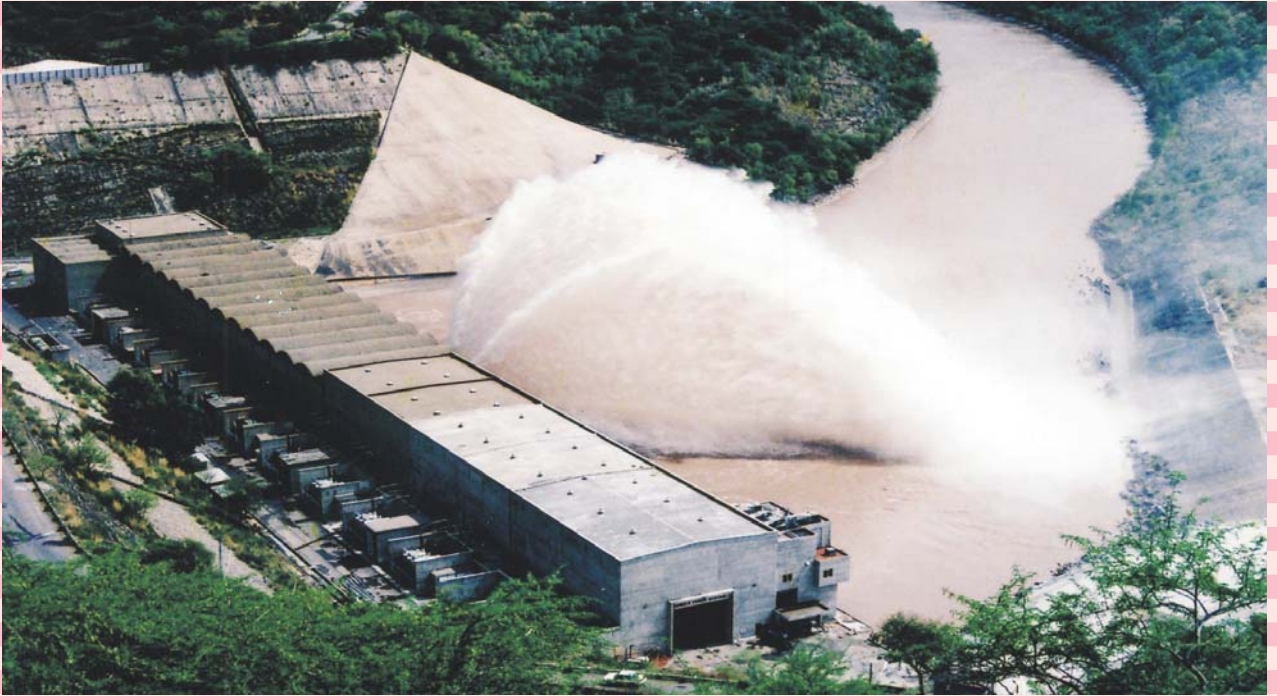
Mangla Hydel Power Station
