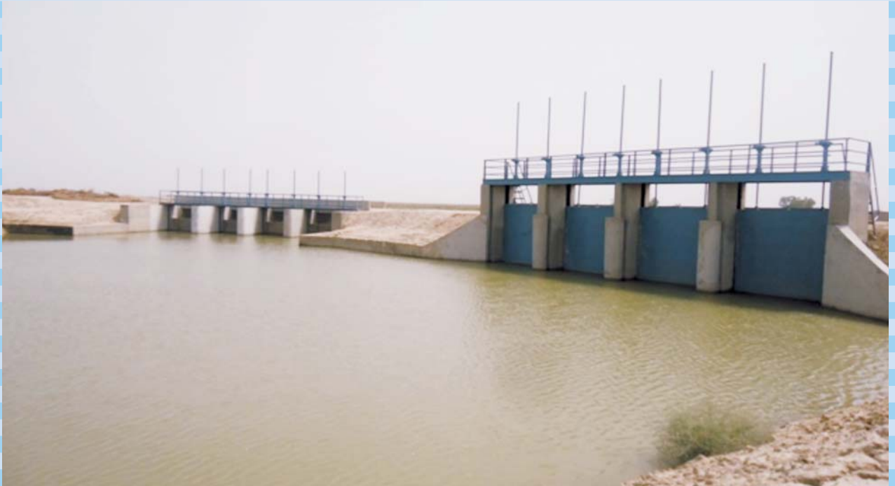
View of RBOD-III Complex Structure at Mero Khan Zero Point
