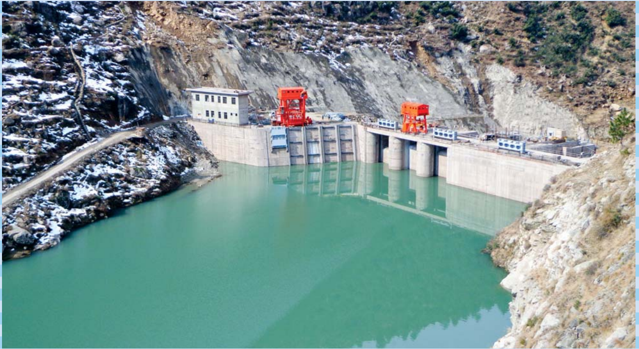
Weir of Allai Khwar Hydropower Project
