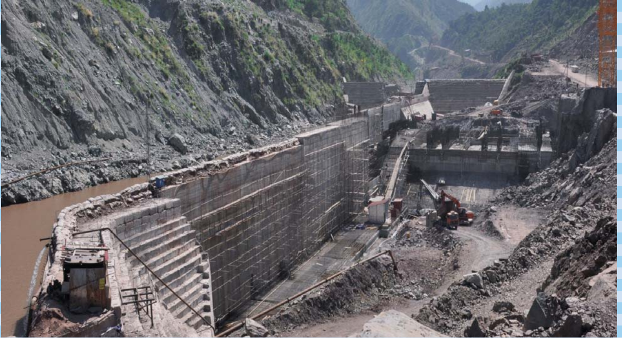
Construction work on Neelum Jhelum Hydroelectric Project
