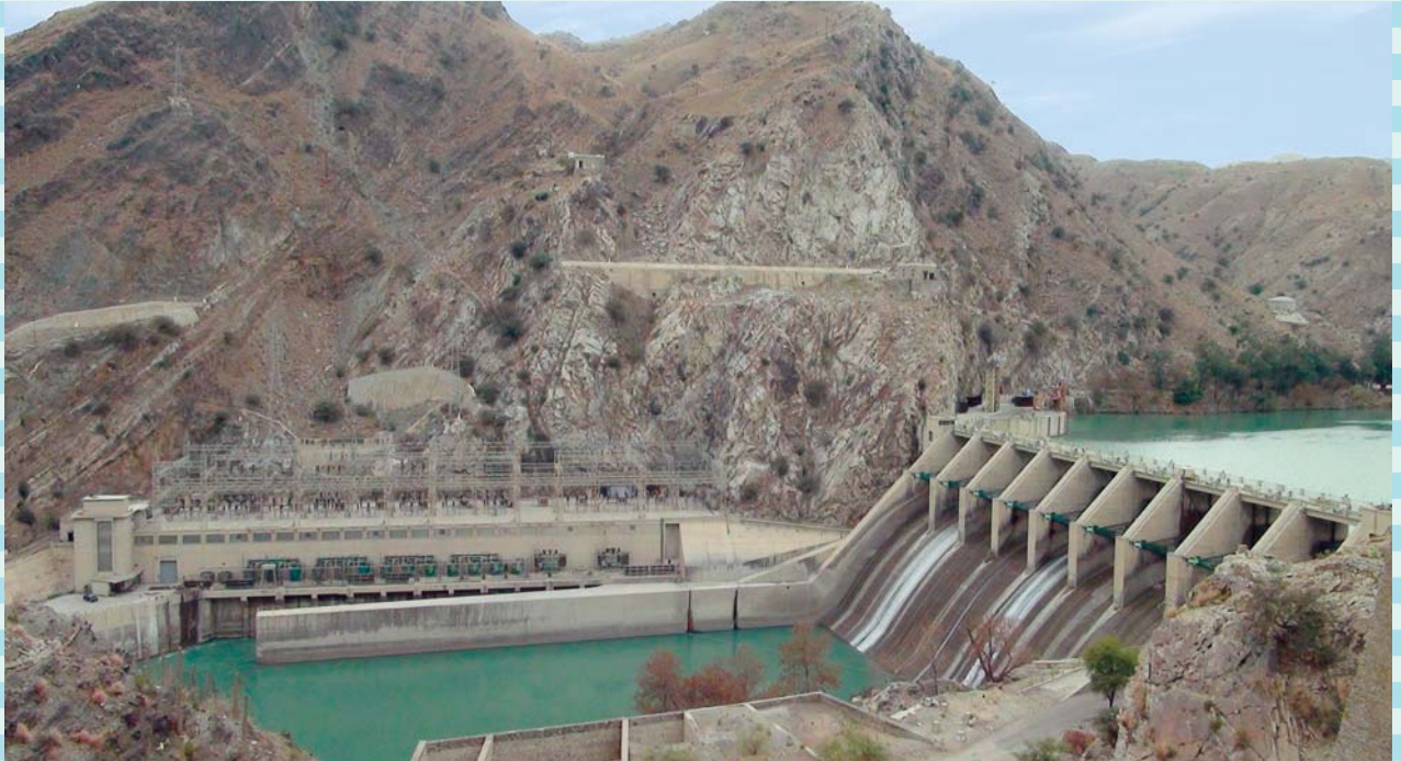
Warsak Hydel Power Station and Spillway
