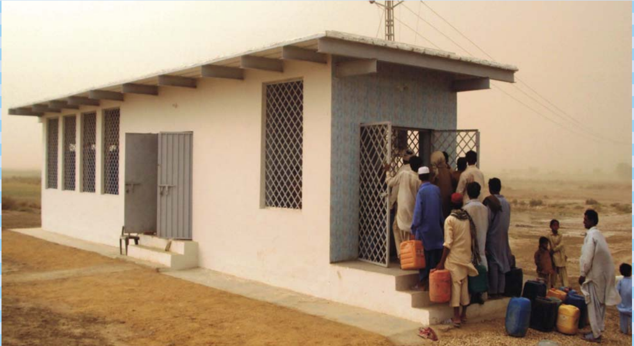
View of Water Treatment Plant Installed at Manchar Lake
