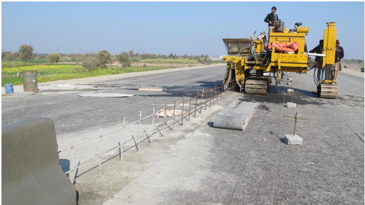
Figure 9.4 Heavy Machinery used During Construction
