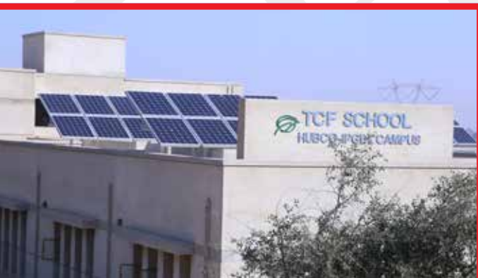
Solar panel installation at TCF school in Hub (Hubco)
