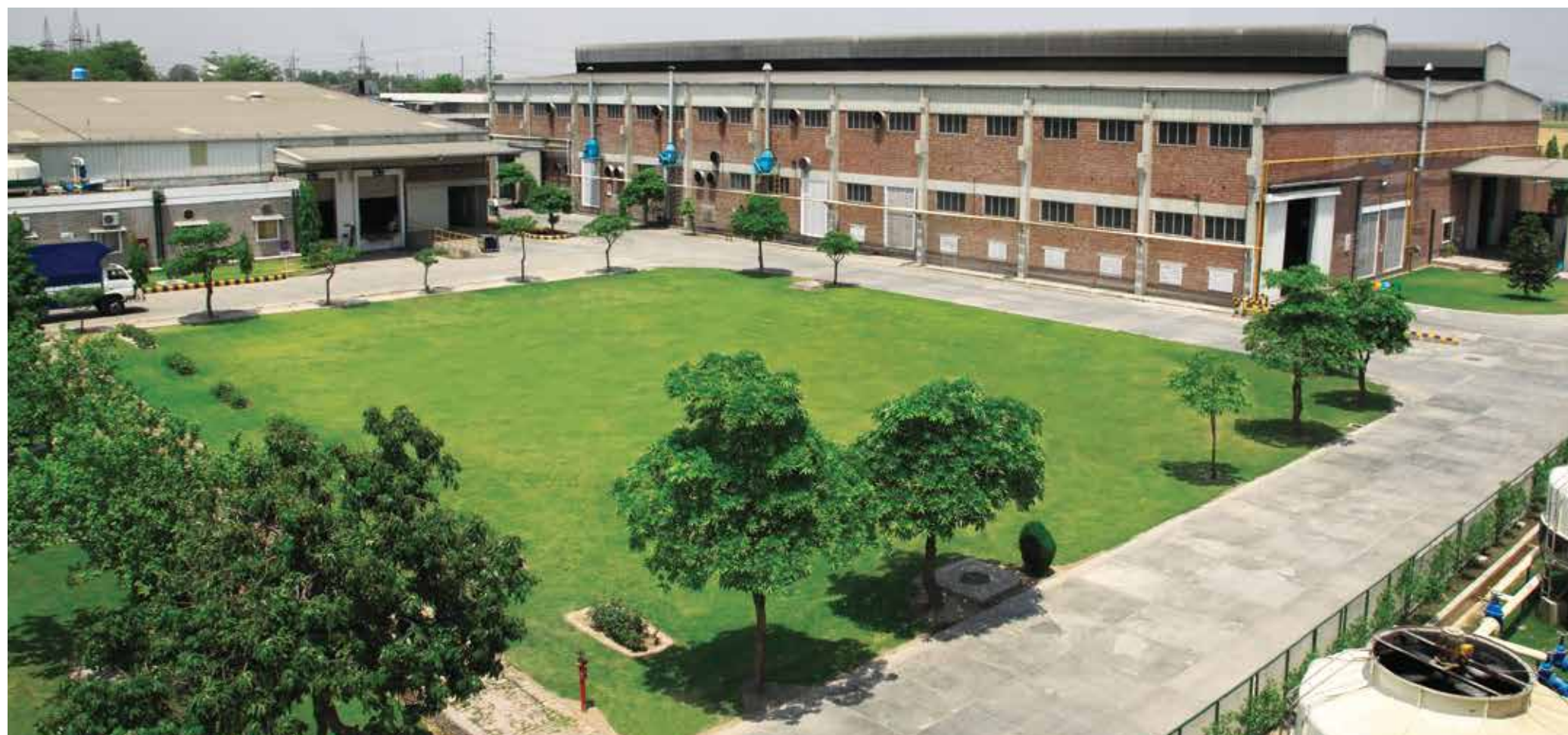
Inside view of Sheikhupura plant
