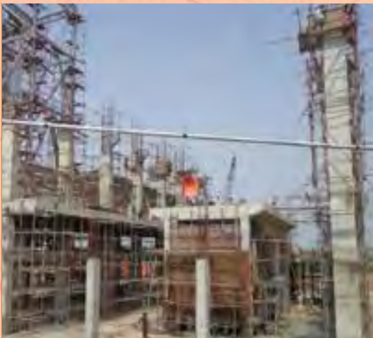
Current view of Coal Fired Power Plant
