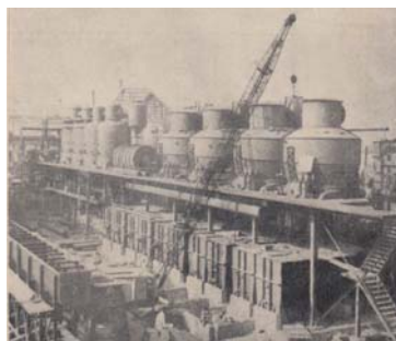
Erection and installation work of complete plant at factory site in 1965.
