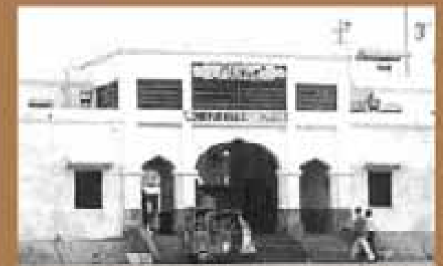
Built circa 1950, the Mirpurkhas Railway Station.
