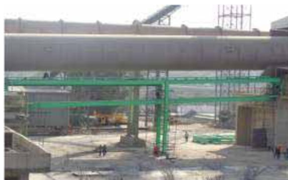
Erection Work in Progress
