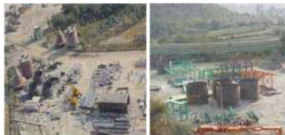
Mechanical Fabrication work in progress
