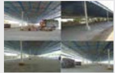
Inaugration of newly constructed Tyre and Store shed at DGK plant.
