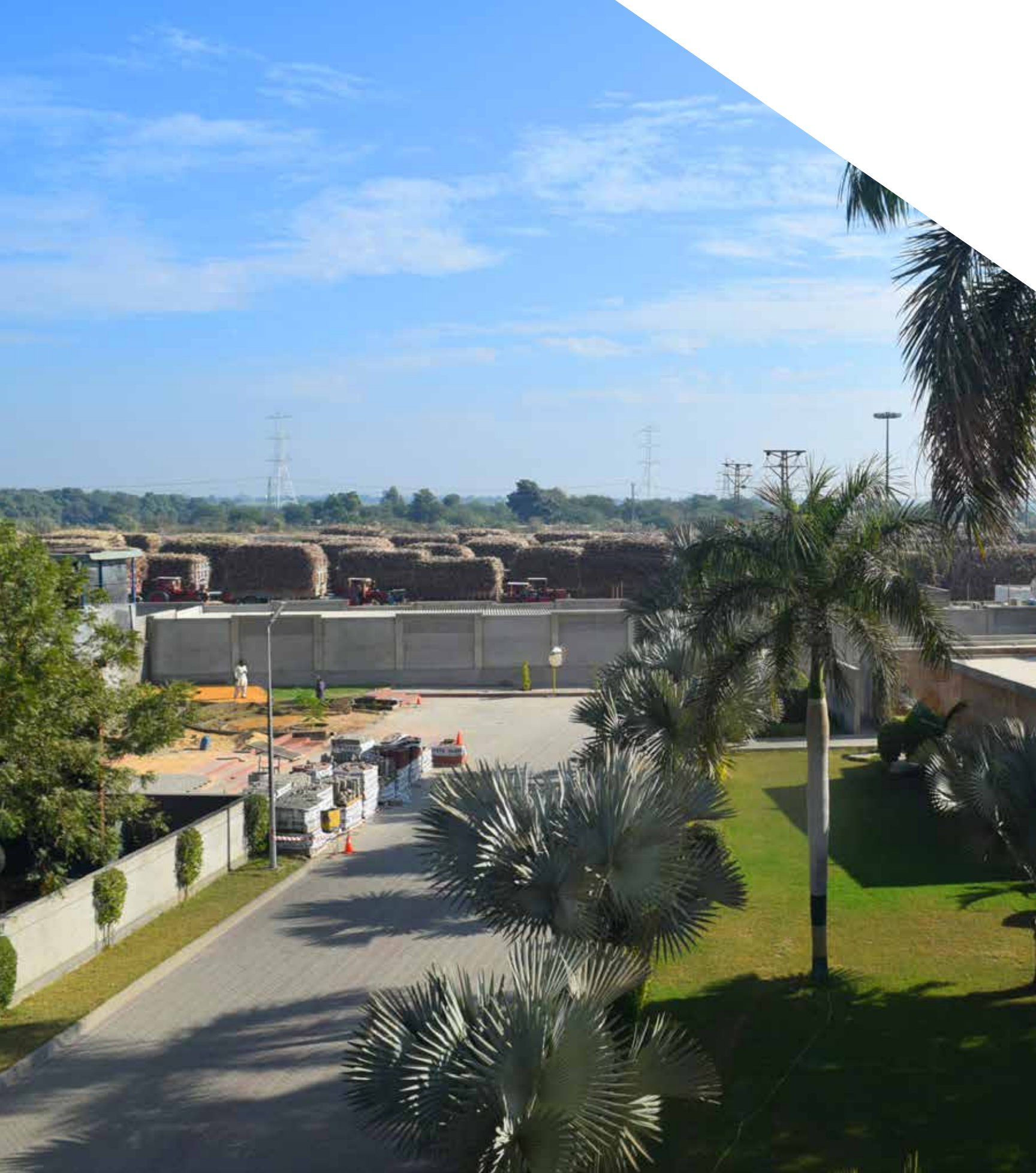
Our newly renovated mill entrance and new outer cane yard across the boundary.
