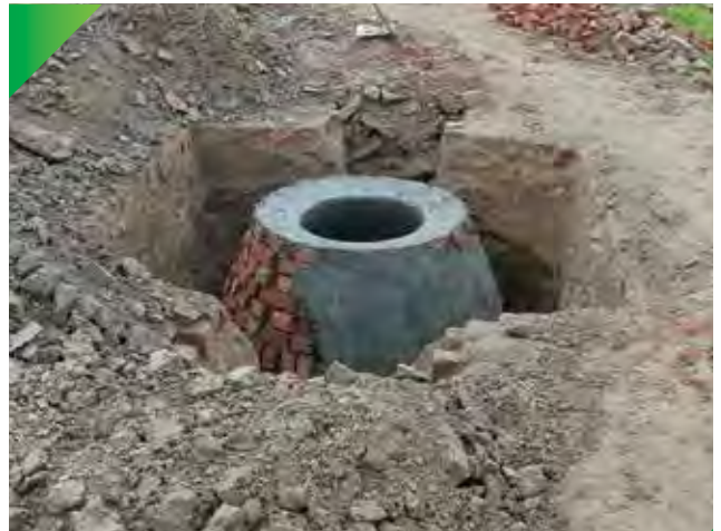
Construction of the underground Sewerage Pipeline
