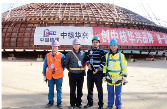
PNRA Inspector at C-4 Dome Placement Activity
