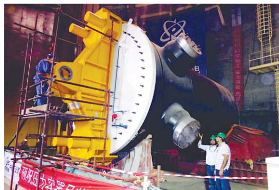
PNRA Inspectors Conducting Inspection of C-3 RPV at Chashma Site
