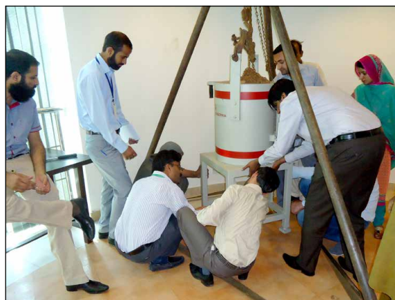
Installation of Gamma Spectrometry System at NEMP Laboratory, Islamabad
