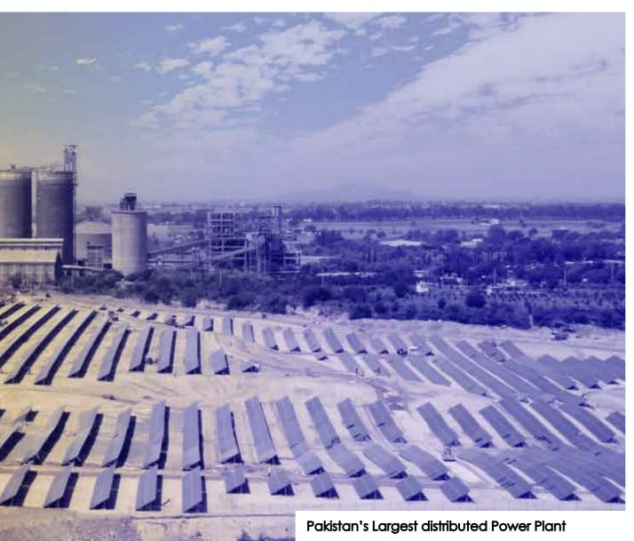
The FCCL 12.5 MW Solar Captive Power Plant in Fateh Jang, Attock District is Pakistan's largest distributed Solar Power Project. The annual energy production of around 19,360,000 kWh translates to the carbon reduction impact of 484,000 trees.
