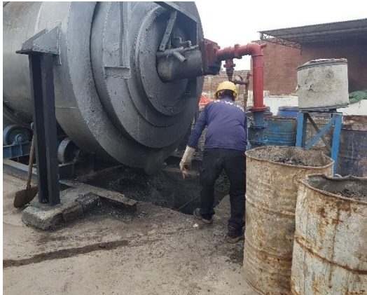
Ash Removal from the pit
