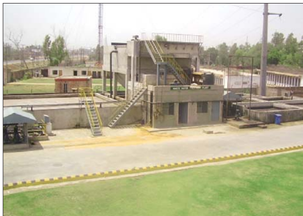
Waste water treatment plant
