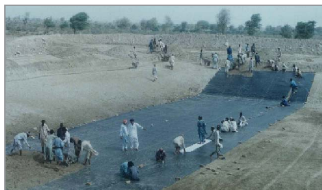
Geo membrane to prevent water seepage losses.
