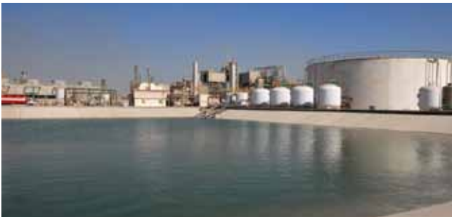
EPCL Raw Water Pond
