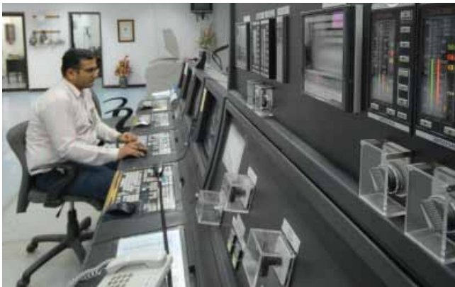
EPCL Central Control Room at Plant Site
