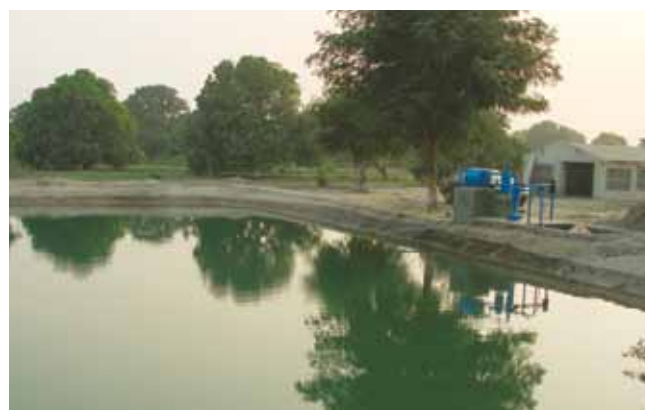
Agricultural pond lined with geomembrane in Rahimyar Khan
