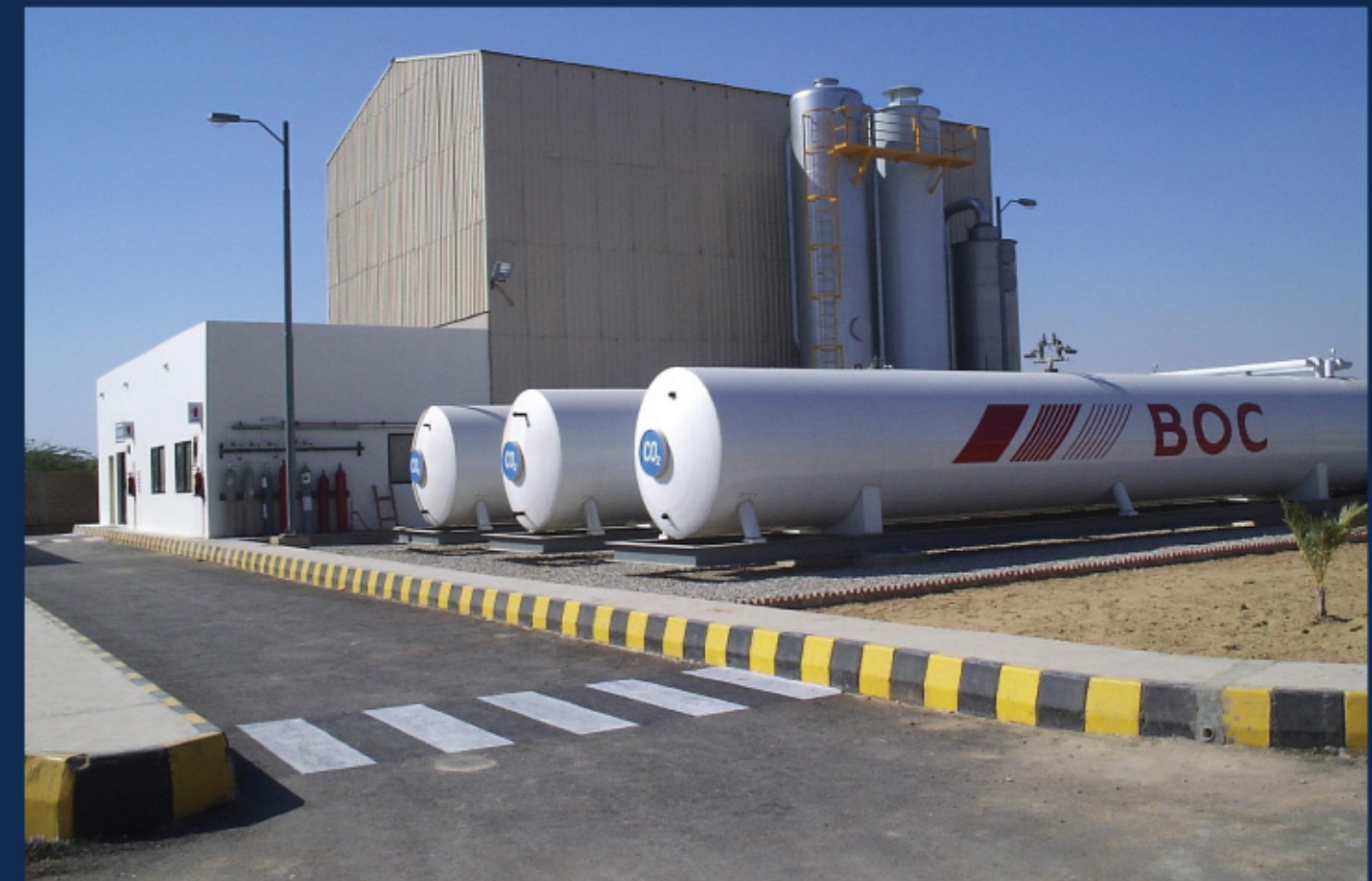
A view of the new 23 TPD CO 2 Plant at Port Qasim
