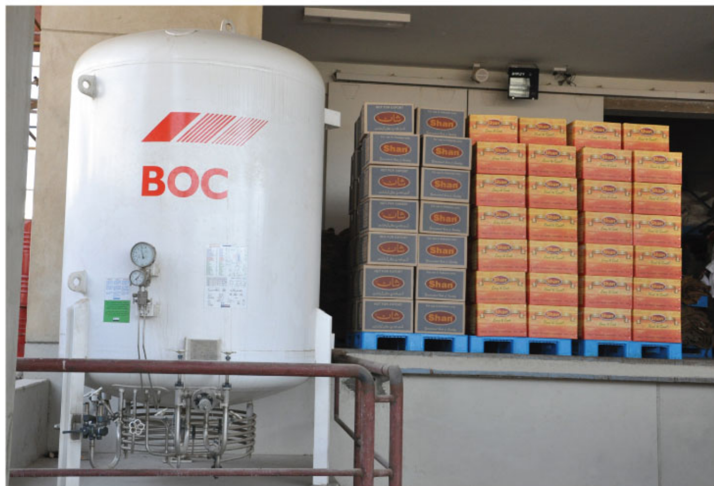
Liquid Nitrogen application in a renowned food processing plant in Karachi
