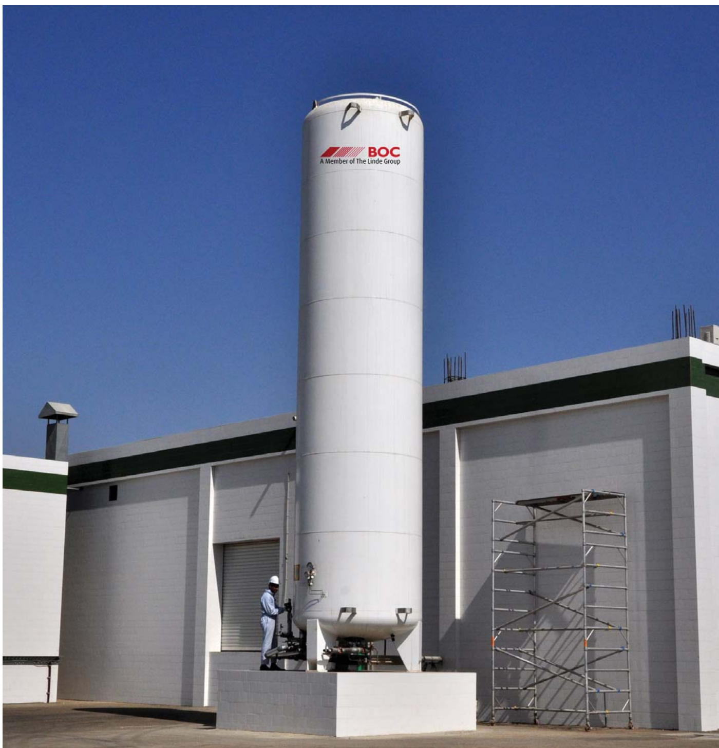
Installation in progress at a new customer in food sector
