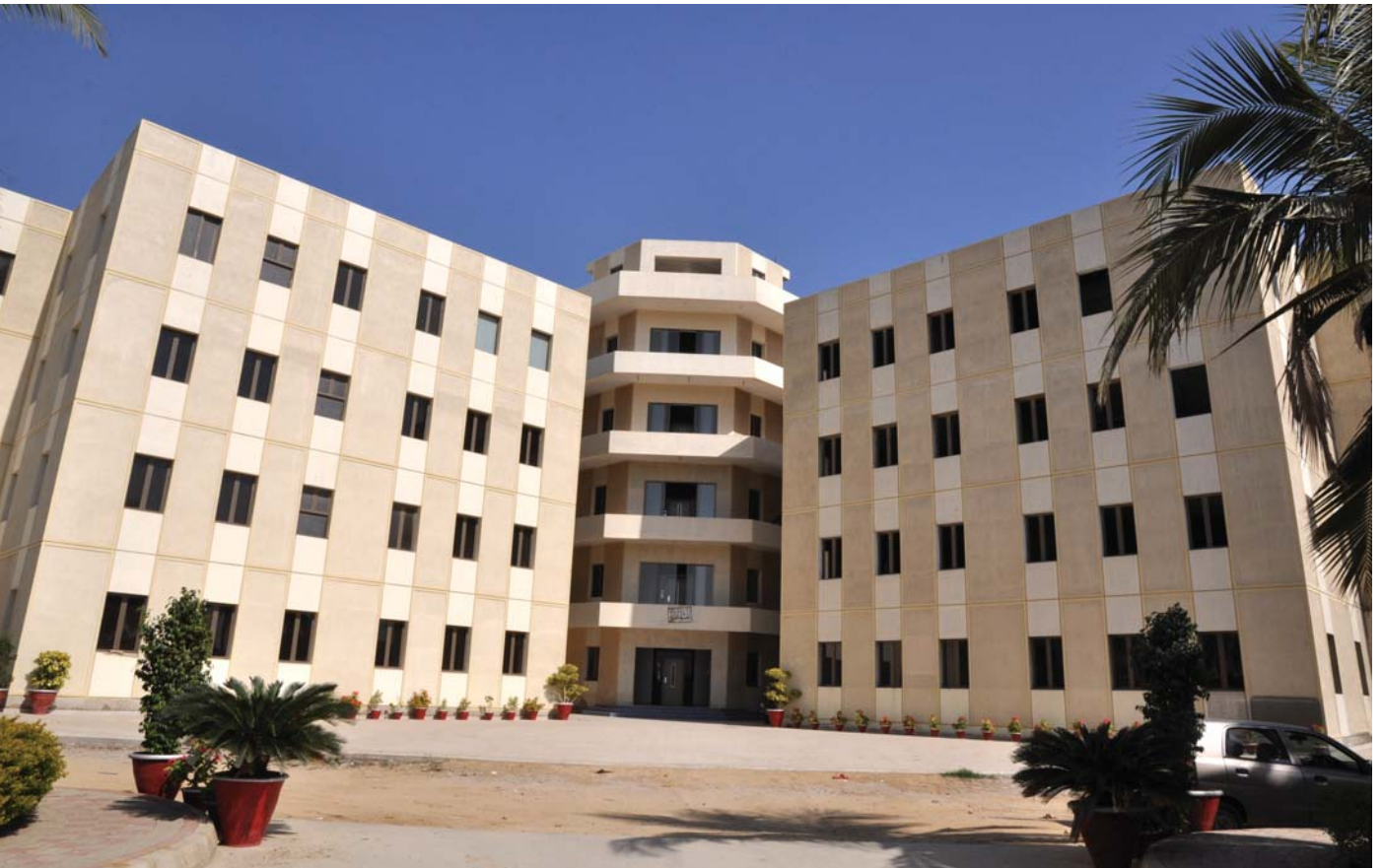
BOC Healthcare successfully accomplished installation of Centralized Medical Gases Pipeline System at a newly constructed four hundred bedded Mehrun Nisa Hospital in Karachi
