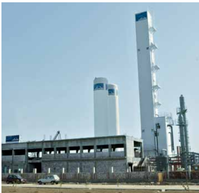
Sundar ASU Plant nearing completion
