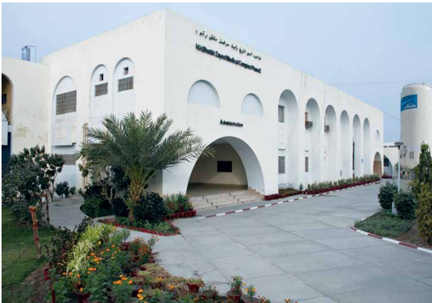
Linde installed a 10 KL tank for bulk liquid medical oxygen at Shiekh Zayed Medical College and Hospital, Rahim Yar Khan
