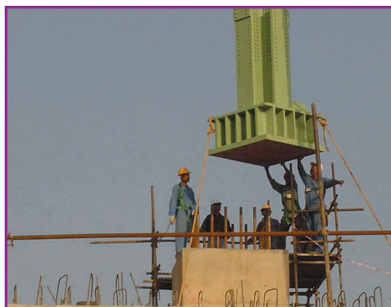
Erection of Pre-heater tower
