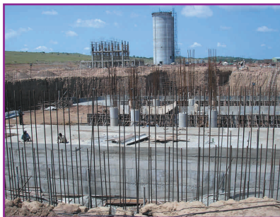
Clinker Storage Yard
