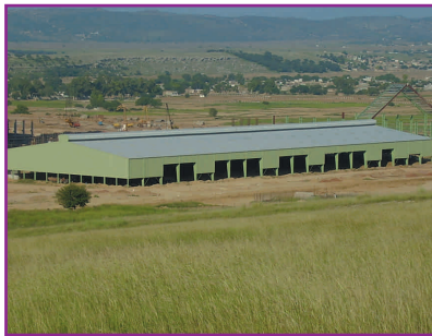
Coal Storage Yard
