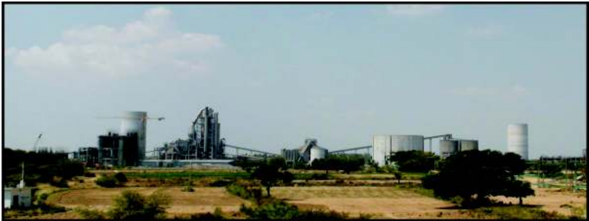
Existing and Under Construction New Line of Production
