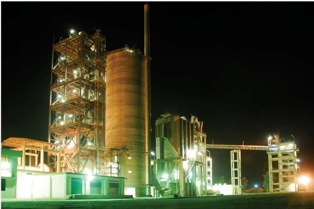
View of newly commissioned white cement dry process plant of 500 tpd
