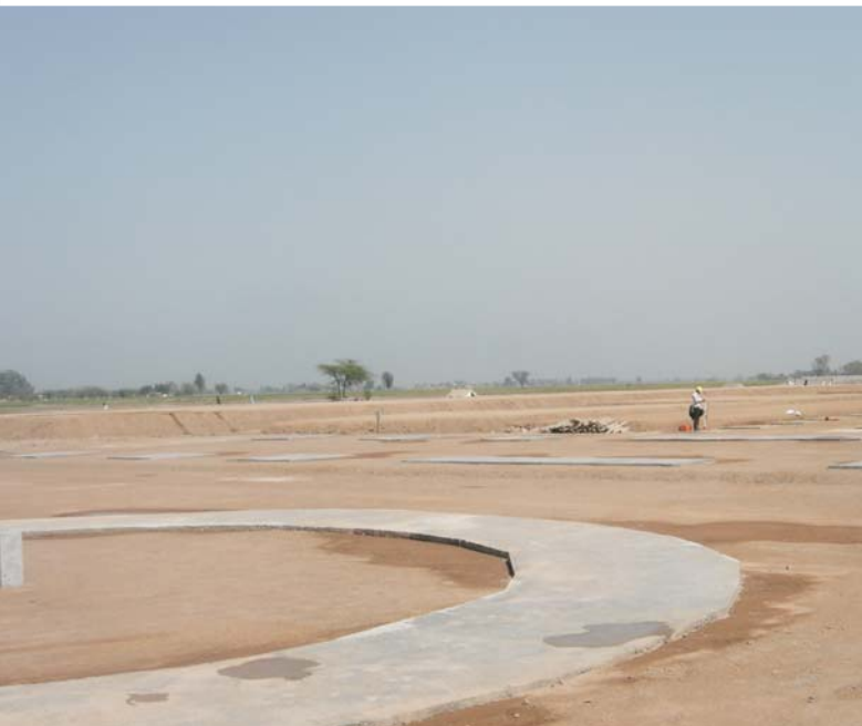
Lean concreting work at the Tank Farm
