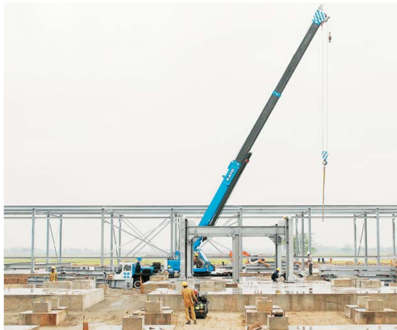
Structural works at the Exhaust Stack
