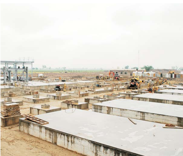
Power House 2 area
