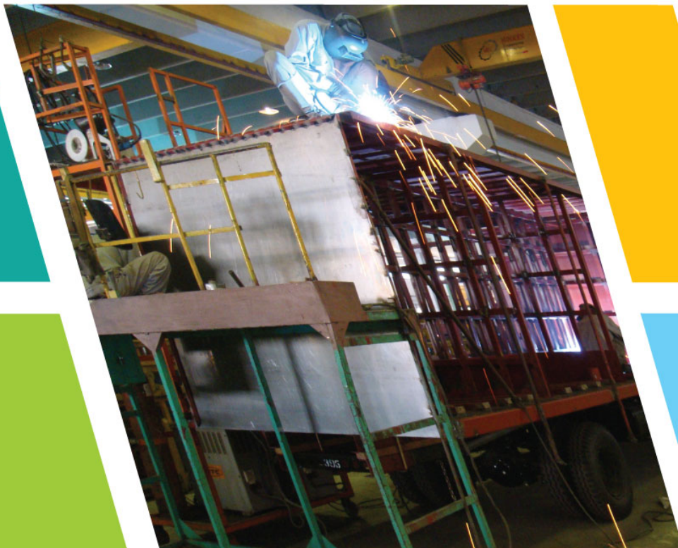
Work in progress at our Body Operation Division
