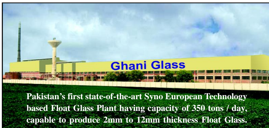
GGL-III SHEIKHUPURA (FLOAT GLASS MANUFACTURING PLANT)
