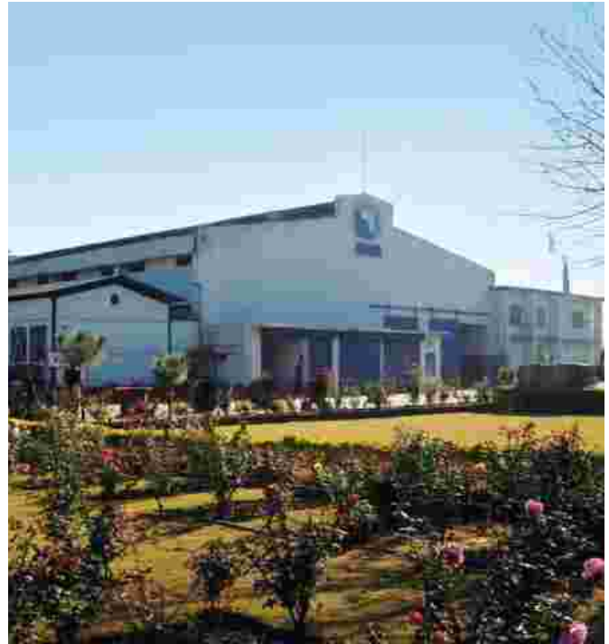
KSB Works Hassanabdal
